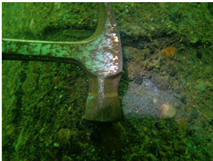
Figure 50. Photo. Typical cold joint after cleaning.
